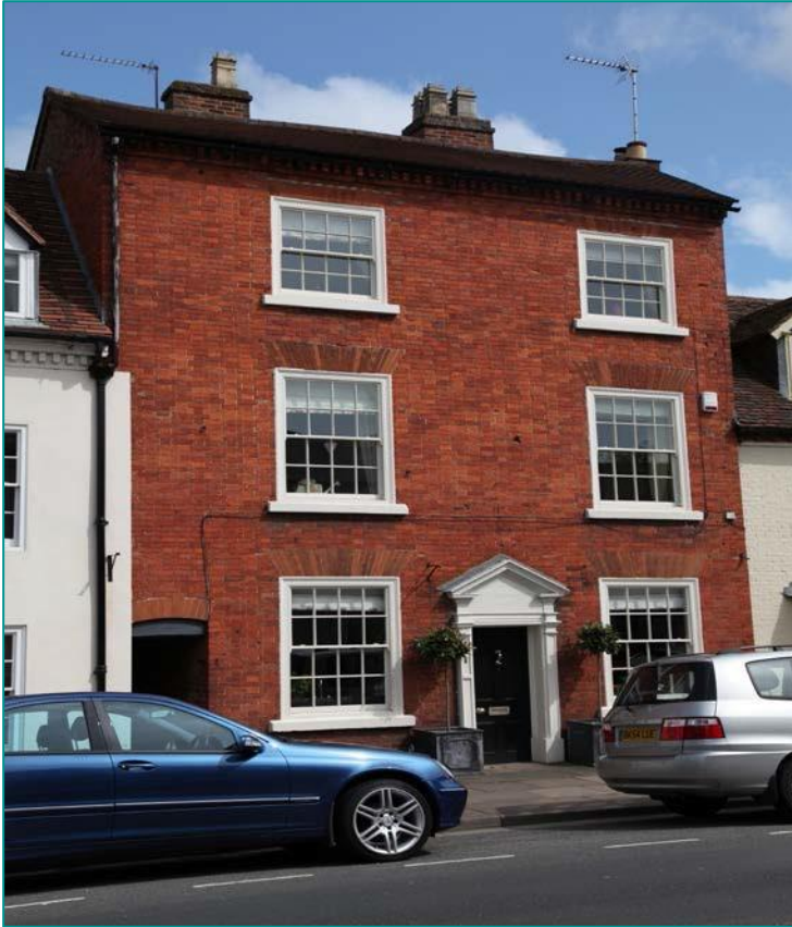
Fig. 2 - Photo of a brick house with rubbed brick flat arch window heads in Henley-in-Arden, Arden area.
