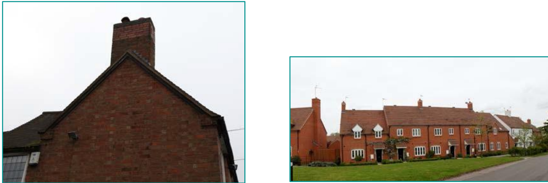
Fig. 11 - Examples of chimney in traditional and new dwellings.
