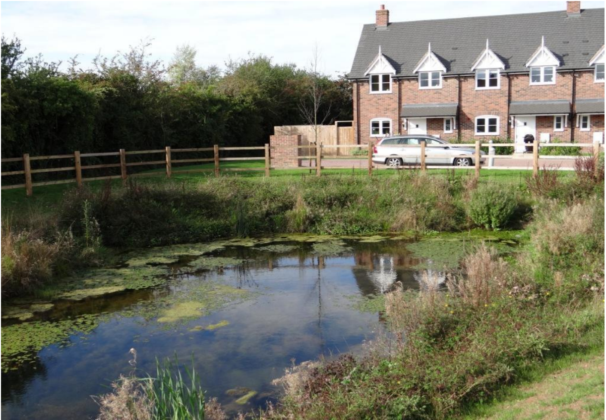
Fig. 2 - An example of SuDS swale, providing multifunctional benefits for residents at Samantha Close, Welford-on-Avon.
