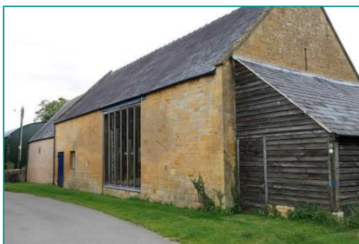
Fig. 9 - Photo of appropriate treatment of midstrey retaining the full height of the opening, Great Wolford.
