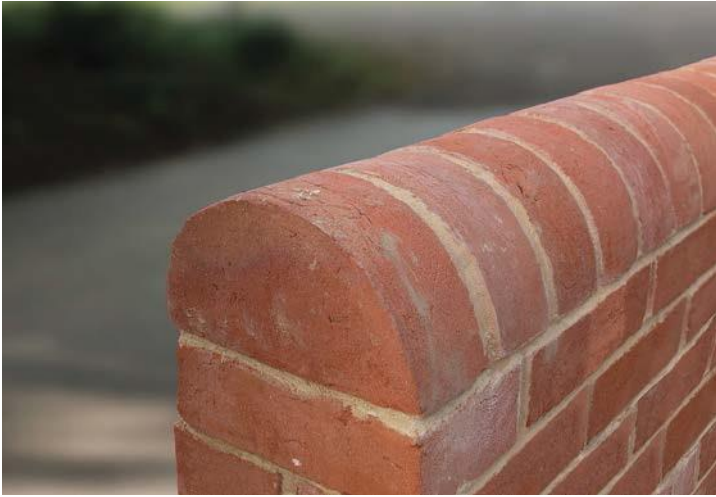
Fig. 22 - An example of a half round copings wall.
