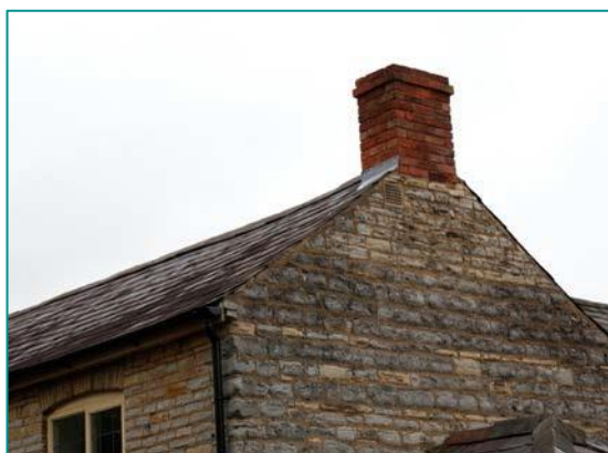
Fig. 10 - Examples of 'wet verge' using mortar to secure the roof tiles
