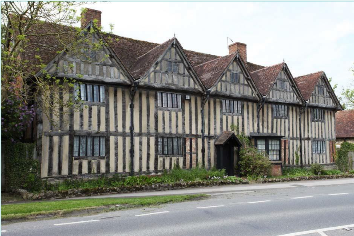
Fig.1 - Photo of close studded timber framed house with rendered infill panels in Long Itchington, Feldon area.
