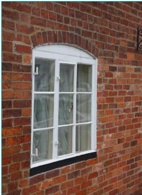
Fig. 5 - A window with a segmental arch head in Alcester, Arden area. Note the arch is made up of headers on edge, a detail very characteristic of brick areas within the District.
