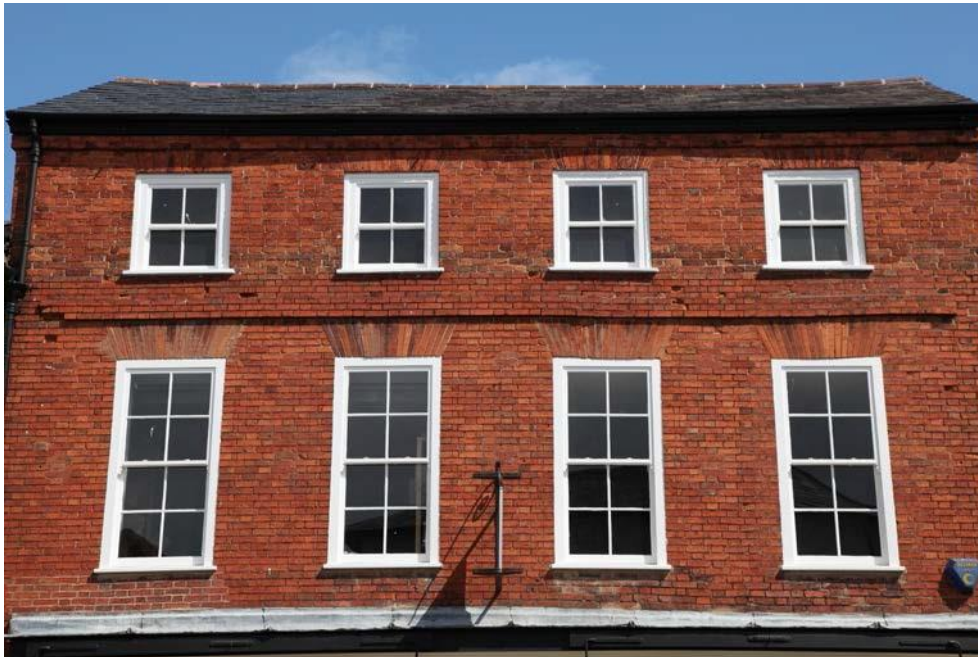
Fig. 4 - Gauged brick flat arches on a house in Henley-in-Arden, Arden area. The openings are vertically aligned and the second floor windows are smaller than the first floor windows.
