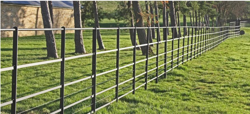
Fig. 23 - An example of estate railings.
