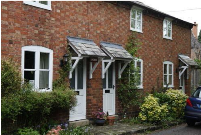
Fig. 6 - Cottages with windows set just below the top plate in Welford-on-Avon, Avon Valley area. The casement windows shown are flush closing as opposed to 'storm proof'.
