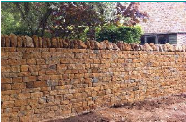
Hornton Stone wall
