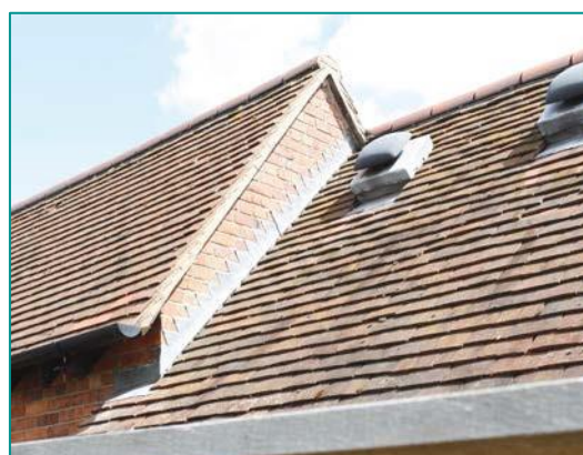
Fig. 10 - Examples of 'wet verge' using mortar to secure the roof tiles
