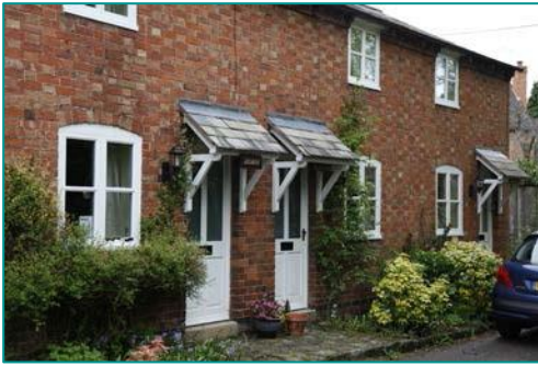
Fig. 13 - Lean to canopies with brackets, Welford-on-Avon, Avon Valley. The roof material is inappropriate in this case as smaller roof tiles are needed.
