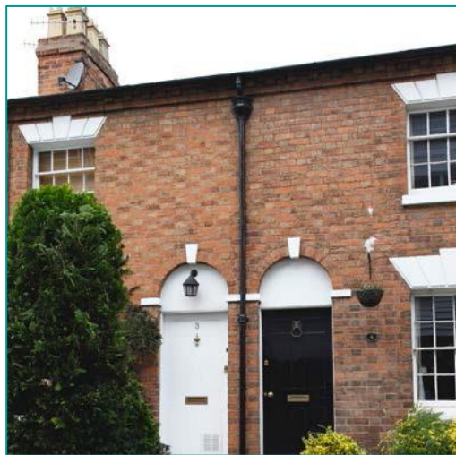
Fig 7 - Render used to create the effect of stone lintels in Wellesbourne, Avon Valley area. The windows have stone cills and sliding sash frames.
